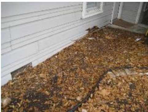
G=Wood to Ground Contact / L=Footing too Low / High Soil Grade
