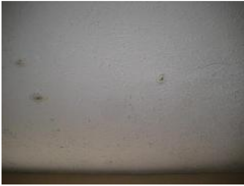
J=Excess Moisture / Water Stains
