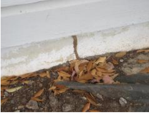
Active Sub-termites on Front of House
