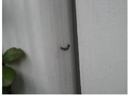
Active Carpenter Ants on Front of House
